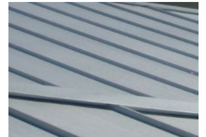
WEATHERED MILL FINISH METAL ROOF
