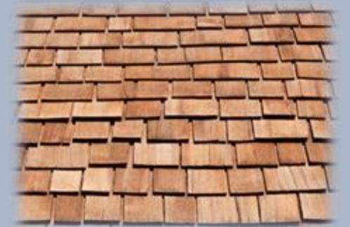
Cedar Shake Roof
